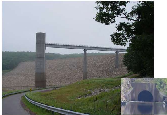
Figure 30: Francis E. Walter Dam located in Whitehaven, Pennsylvania. Concrete outfall structure located on the downstream side of the dam is shown at bottom right.
