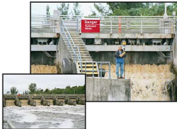
Figure 10: Real-Time kinematic survey of Corps lock and dam project--hand-held fixed height antenna pole.
