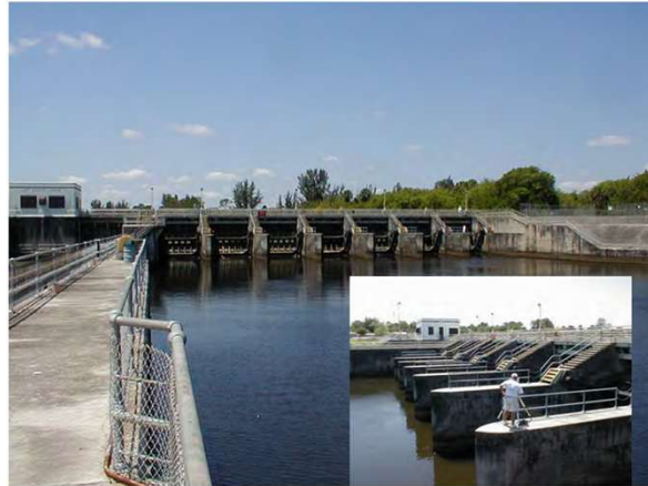
Figure 23: Typical scan location to cover downstream gate structures--instrument set up between 6th and 7th gates.
